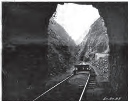
Tunnel Near Tamboque on Oruya Railroad, 9,826 Feet Above the Sea Level.
