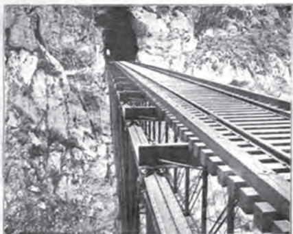
Infernillo Bridge and Tunnel on Oruya Railroad, 10,919 Feet Altitude.
