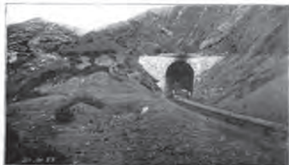
Galera Tunnel, 15,665 Feet Above the Sea Level. The Highest Point Ever Reached by a Railroad.
