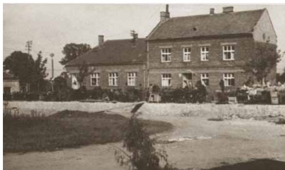
Photo 29 The building of the former telephone exchange and officers' club as they were in 1944
