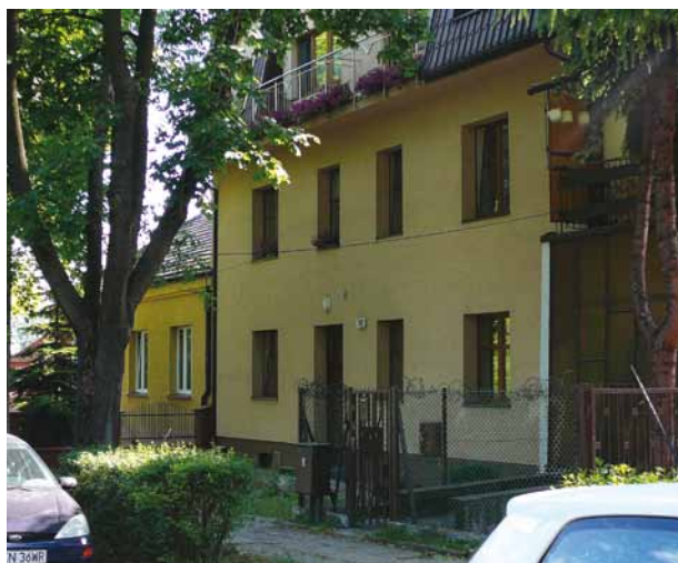
Photo 30 The building of the former telephone exchange officers' club today
