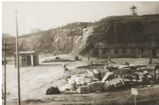
Photo 56 The main quarry within the camp, an anti-aircraft tower above it
