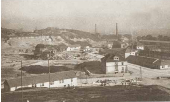
Photo 55 The central section of the camp, a view of the area of the Grey House from the anti-aircraft tower. Barracks 172 at the bottom, further: the ruins of the funeral parlor and the SS- Lazaret . On the right: the Kommandantur and staff's barracks behind the Grey House
