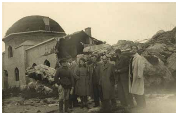
Photo 19 The site of the former camp, 4 October 1945. The first visit to the crime scene paid by members of the District Commission for the Investigation of German Crimes and the Regional Jewish Historical Commission in Kraków (against the backdrop of the ruins of the funeral parlor)
